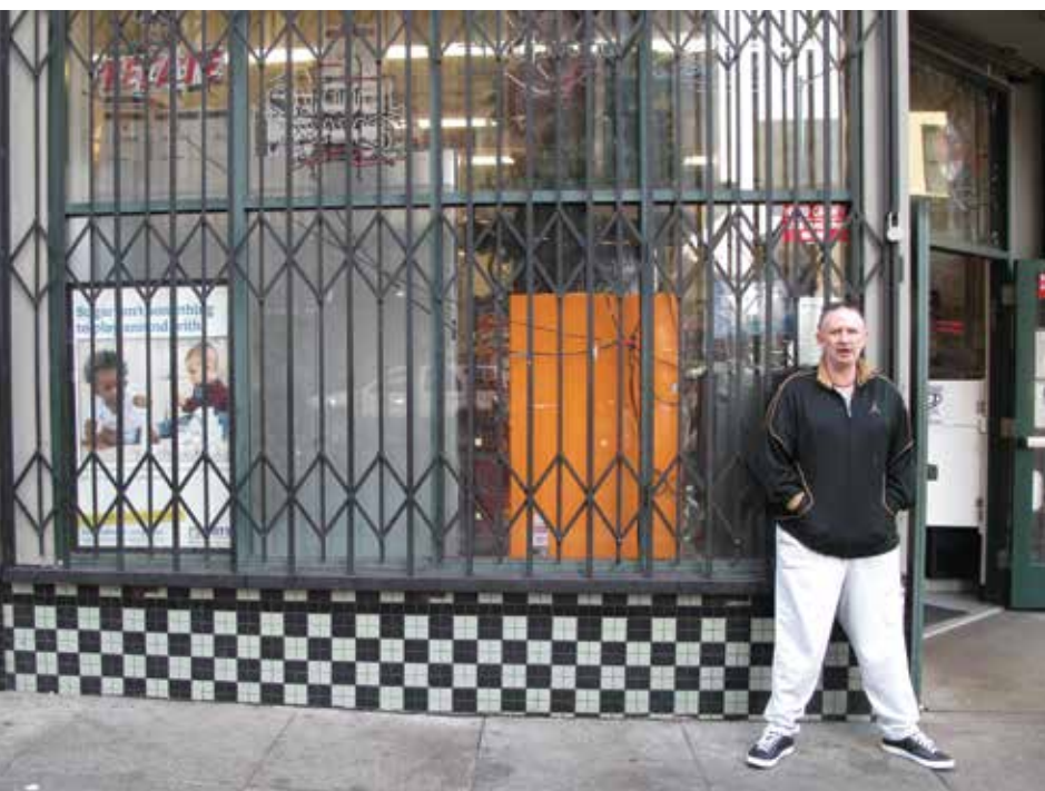
G&H Market , with a passerby standing in front, needs major readjustment, Purvis notes, because of the security gate outside and large refrigerator cases inside.
