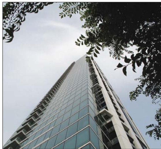
The developer of One Rincon Hill's South Tower paid his fees in full; the North Tower construction is on hold.
