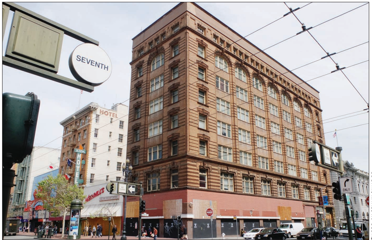
The handsome Grant Building anchors the southeast corner of Seventh and Market. The landlord's heavy hand, helped by the long arm of the law, made working in the historic building's last days cold and miserable.
