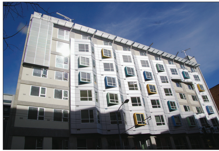
Salvation Army's new building on Turk Street with community center and housing.
