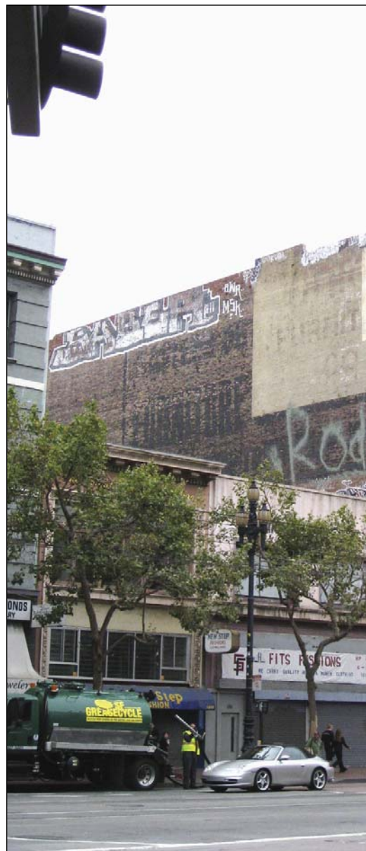
Furniture and Carpets , the store with Greek columns would be a candidate for one or more signs on the street.
