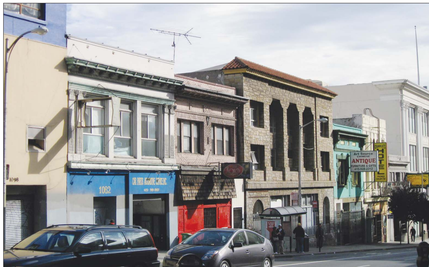
The seven buildings left to right on the north side of Geary all will be razed for the Cathedral Hill medical office building.
