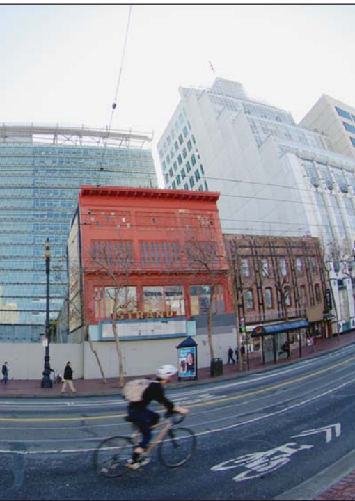
ole left by the demolition of the Embassy Theater, to the right, and the Odd Fellows Hall at far left.
