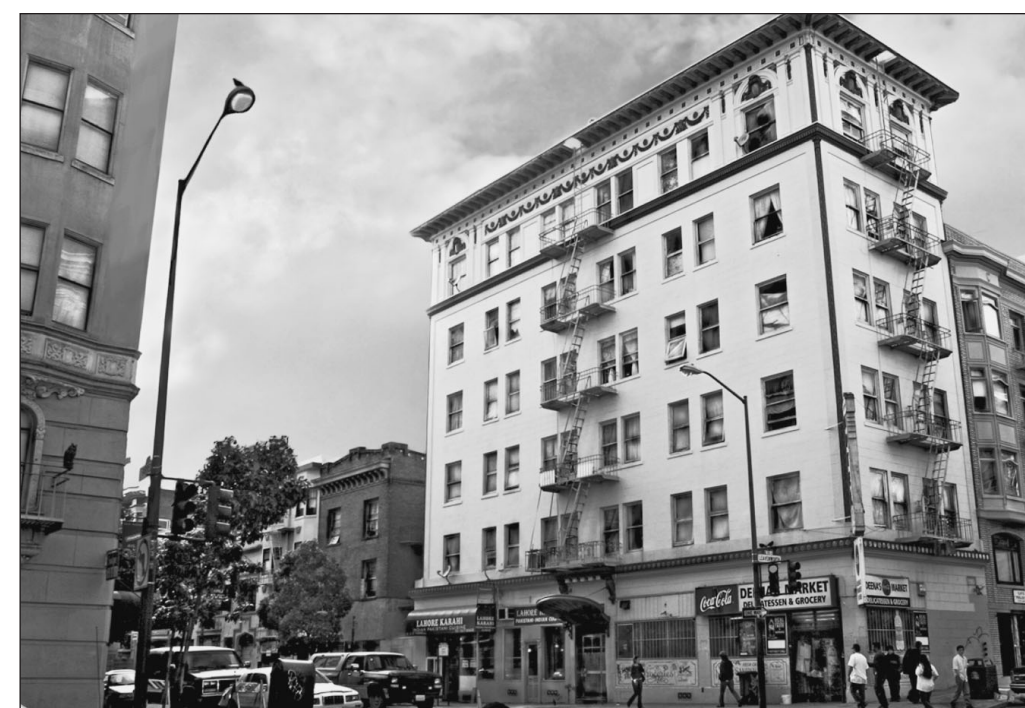
Under the wide projecting cornice of the Admiral Hotel, 608 O'Farrell, are garland reliefs, projecting cartouches above four of the windows, and a belt course that separates the top story.
