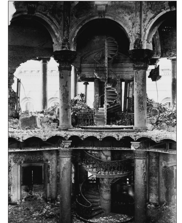
The aptly named Majestic Theatre at 1281 Market St. was turned to rubble.
